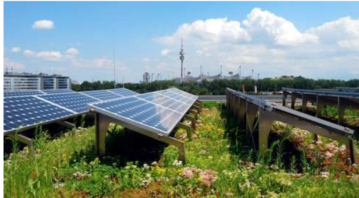
Example of PV roof array
